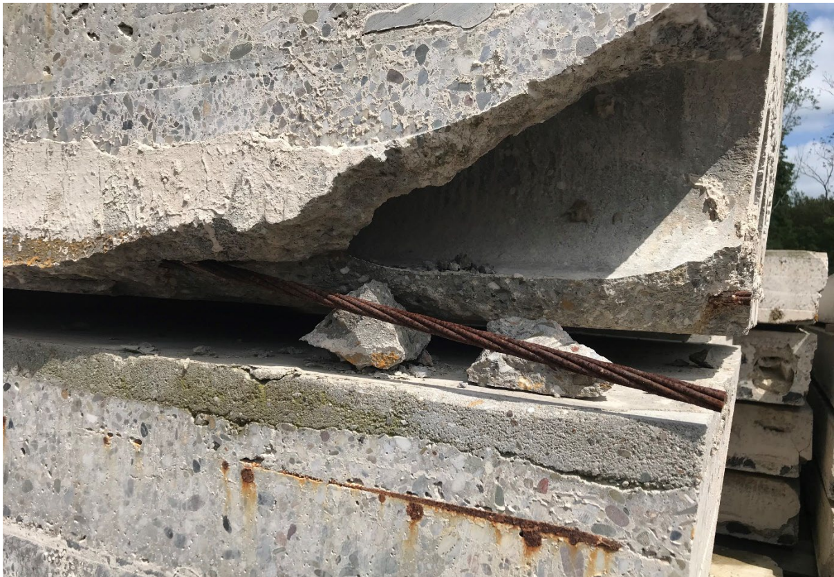
Figure 8. Damage from deconstruction in a hollow-core slab. Photo © TAU/Jukka Lahdensivu.
