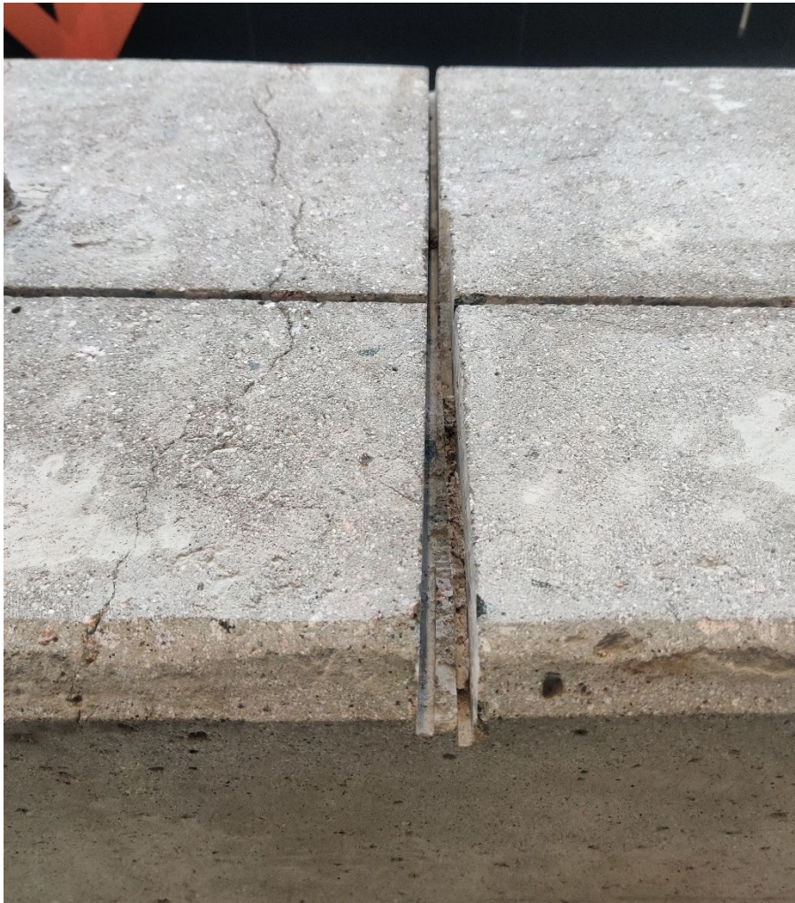
Figure 13. Sawing grooves from deconstruction on top of a beam. Photo © TAU/Aapo Räsänen.
