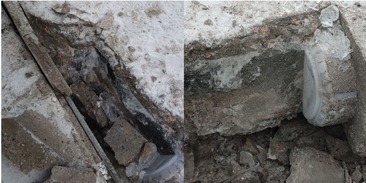
Figure 10. Damage in a hollow-core slab from freeze-thaw exposure during deconstruction. Photos © TAU/Emmi Salmio.
