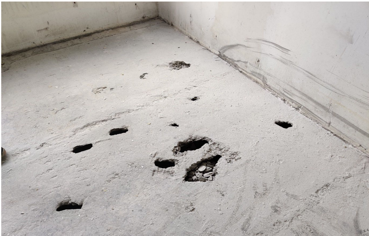
Figure 6. Holes on top of the hollow-core slabs from removing screed in deconstruction stage. Photo © TAU/Aapo Räsänen.
