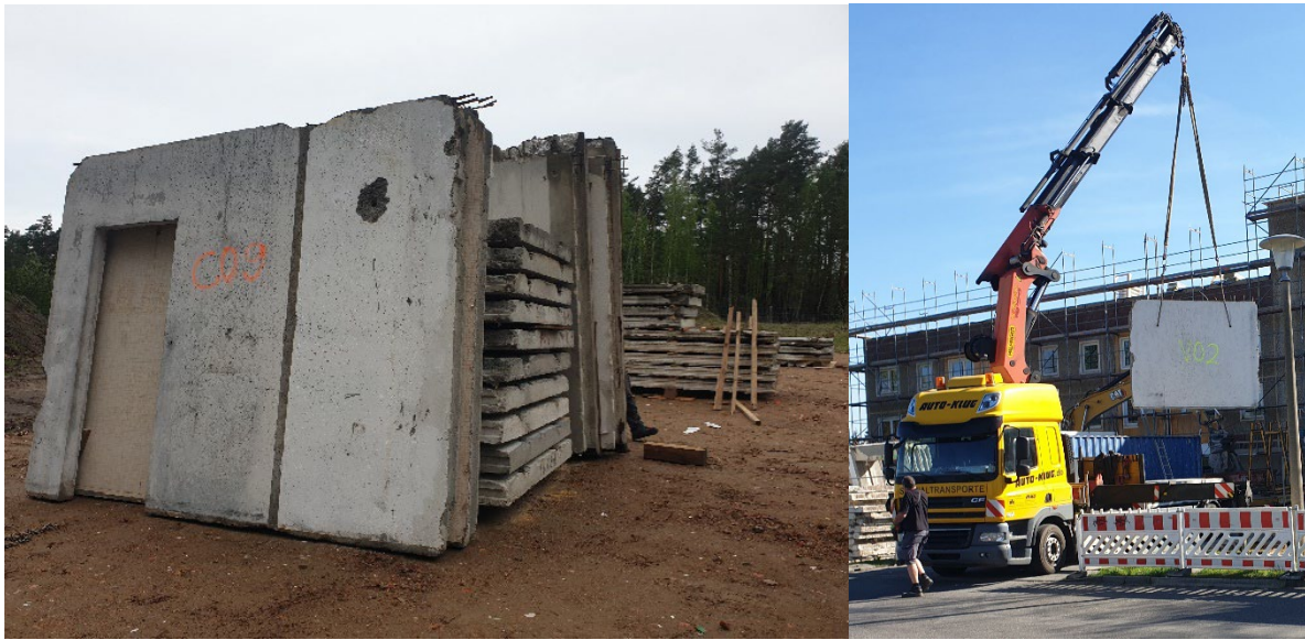
Figure 7. Damage in a wall element cause by deconstruction and lifting. Photos © BTU.
